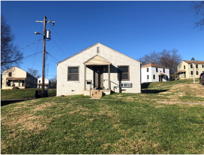
C-12 North side and adjacent, taken 1/11/2022
