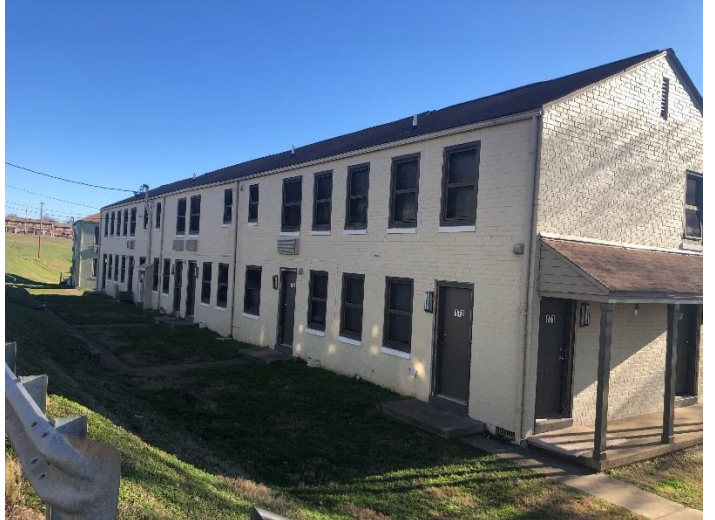
North side of A-50 looking southeast, taken 1/11/2022
