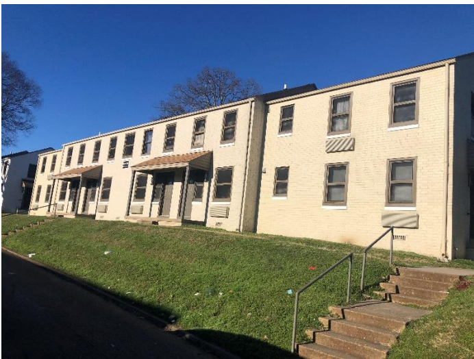
A-50, two story eight-plex taken 1/11/2022
