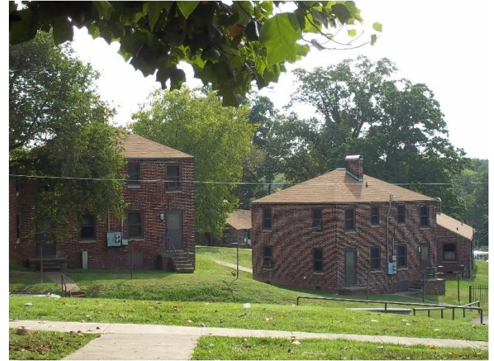
Two story units taken 7/22/2010 prior to renovation
