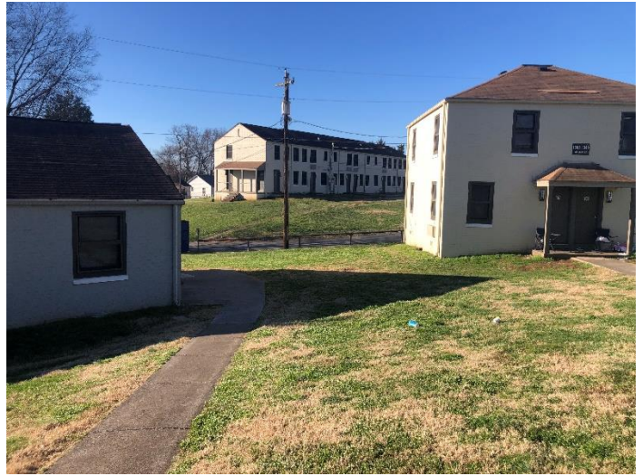
C-12 and adjacent units, taken 1/11/2022
