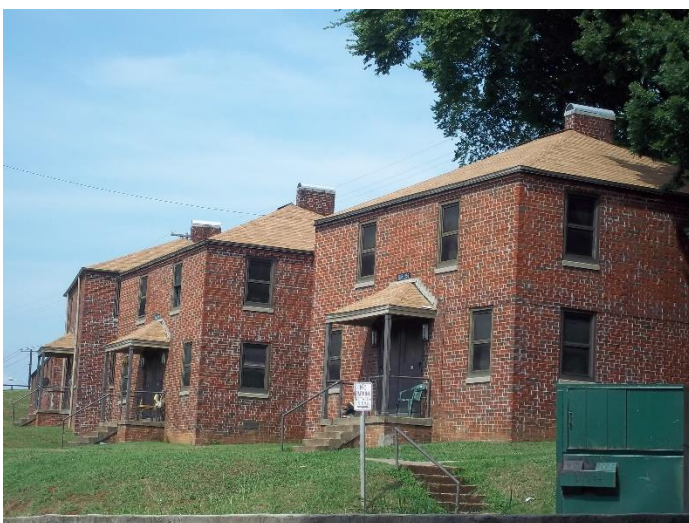
Two story units taken 7/22/2010 prior to renovation
