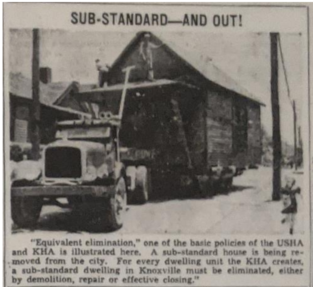
A substandard tenement house being removed. Knoxville New Sentinel 8/4/1940
