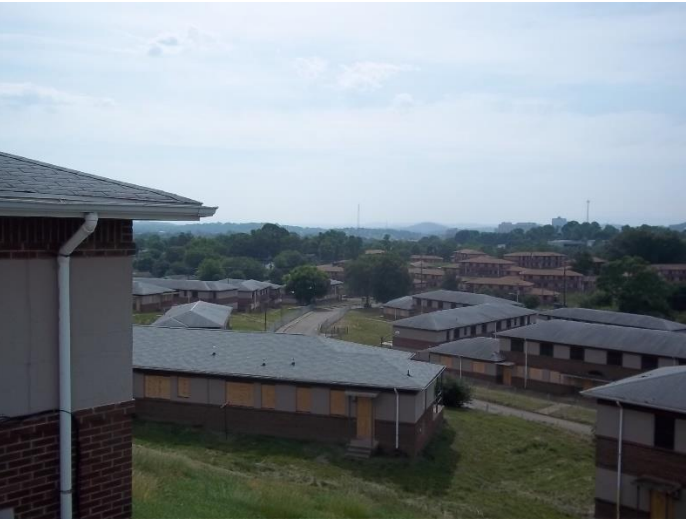
1953-era buildings prior to demolition, taken 5/24/2011
