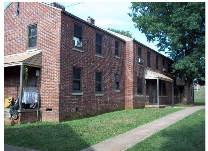
Two story eight-plex taken 7/22/2010 prior to renovation
